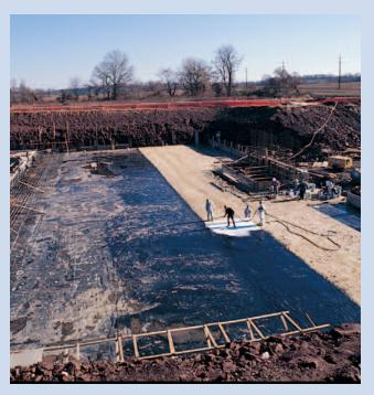
CIM is easily applied and adheres permanently to all surfaces, from soil to concrete to ashpalt.
