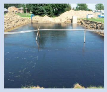
CIM is suitable for below-grade waterproofing applications where ponding water may be present. It is also extremely tough, and no protection board is required.
