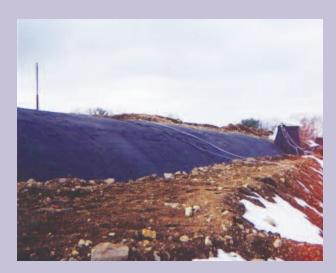
n 80-year-old potable water reservoir had many leaks and cracks. The owners were looking for a coating that could repair the cold joints and the damaged concrete.
